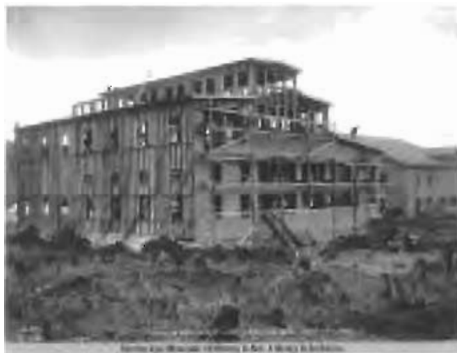
Coal Washing Plant, Oct. 1921 Photo found at http://vilda.alaska.edu
